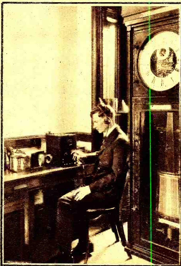
Time Signals from Other Radio Stations Throughout the World are Received at the Naval Observatory and Comparisons Made.
